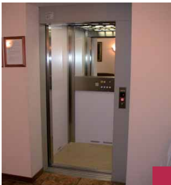
Installation in a hotel (Russia), car with skin plate panels, push buttons and car profiles in stainless steel, half wall mirror.
