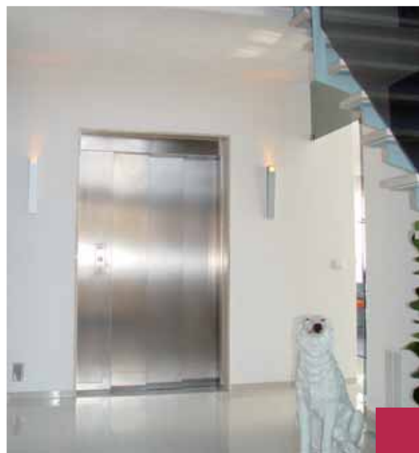
Installation in a private house (The Netherlands), automatic 3-panels telescopic door and stainless steel finishes.
